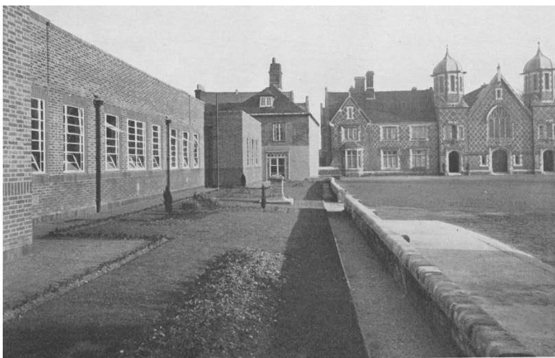
NEW BUILDING AND MAIN BLOCK.
