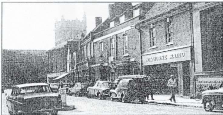
ALWAYS IN VIEW: One of the capped towers
